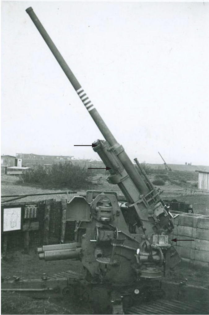
Figure 3. 7.5 cm Flak M 36 (f) gun in German use. Note the Formstein -walls, which remains can be spotted in Figure 1 too. Arrows indicate the (possible) found parts (source: Axis History Forum (2011)).
