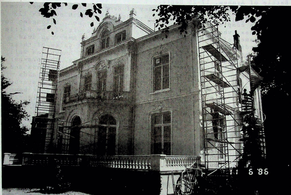
The Hartenstein in scarfolding during painting of the exterior walls. (Photograph: B. de Reus).
